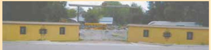
Bill Swets set up 2 schoolbus storage sheds behind his ranch. The side of each bus that faces the road is “dressed up” with hardboard siding and homecrafted decorations.
