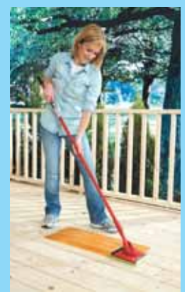
Sprayglide wheel glides along deck to keep pressure washer wand from gouging the wood (left). Shur-Line stain system holds 1/2-gal. of stain or sealer to treat deck boards.
