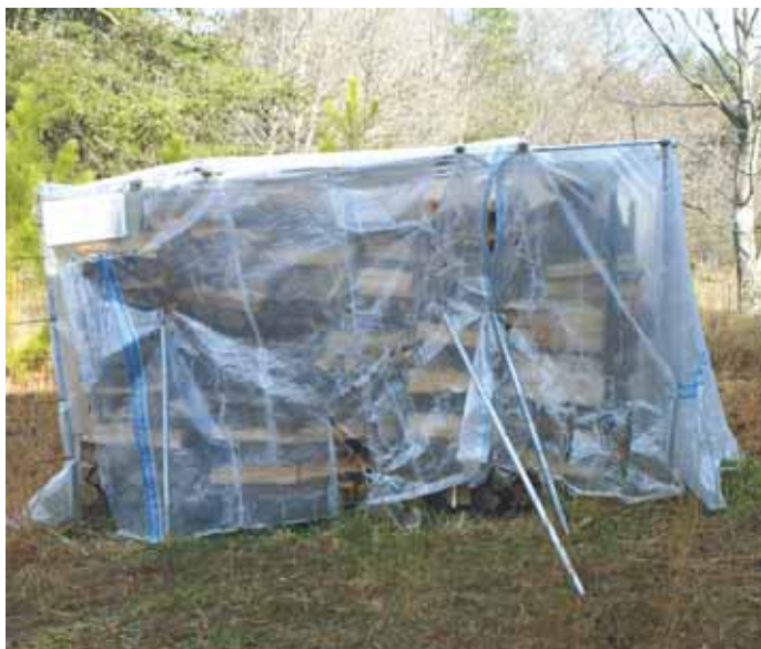
Solar kiln is made from clear reinforced plastic attached with cable ties to a metal tubing frame. Note vent at top left.
