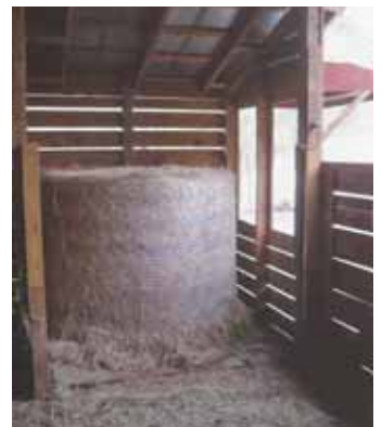
Bale is loaded into feeder from inside the barn. There are 2 large feed openings to the outside.
