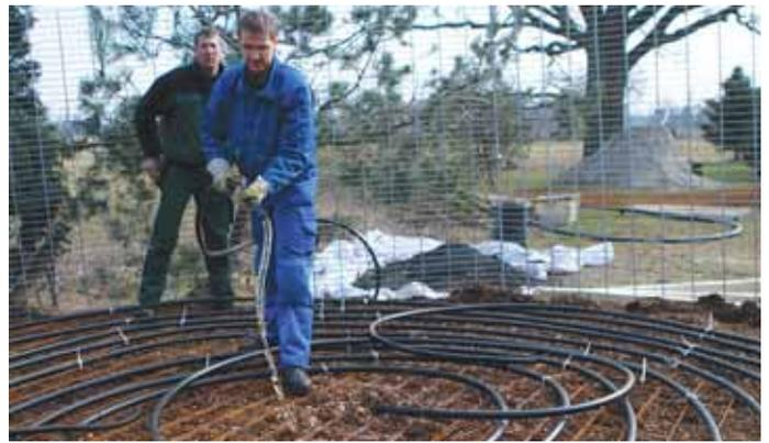
With a circulating pump as the only moving part, the compost heater can last up to 24 months, providing heat and up to 80 percent of the hot water for a 1,500 sq. ft. home.
