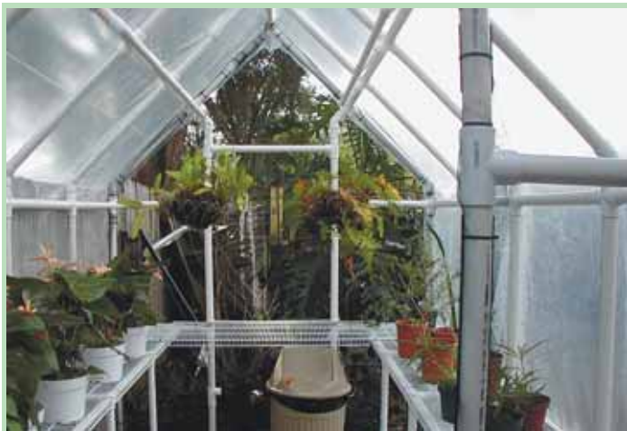
The interior of this greenhouse was made with pvc pipe and fittings from Circo Innovations.
