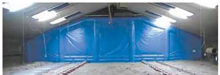
Inflatable "air wall" seals off one end of Jon Steenbeek's 400-ft. poultry barn.
