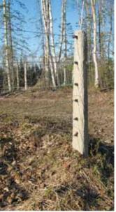
Concrete electric fence posts save Bernie Willis money compared to treated wood posts. Plastic insulators are secured to rebar inside the post.
