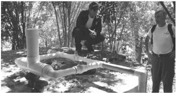
In Nicaragua, engineers created a water chlorinator out of pvc pipe that delivers a controlled dosage of chlorine tablets.
