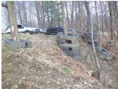
To save trees on worksite slopes, Paul French cut part way through some truck tires and then stacked them around each tree. He then backfilled around tree.
