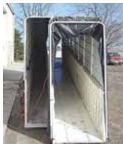
Chute consists of a 32-in. wide walkway for pigs with an 18-in. walkway alongside for people (left). Load-out area is equipped with a 3-panel door.
