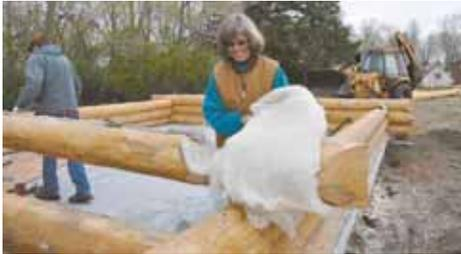
Dee insulates between logs with wood batts and roping.
