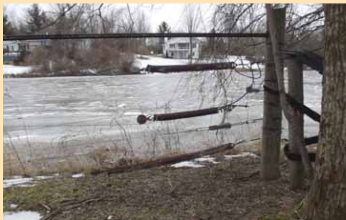
Recycled garage door springs are attached to high tensile fence wire. During spring floods, the springs stretch to keep ice chunks from breaking wires.
