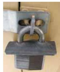
Rubber "umbrella" prevents moisture from entering lock. It has 2 holes in it, spaced to match lock's shackle.
