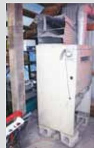
space, which is about 40 ft. away. We cut and bend corrugated metal and anchored it above the furnace fan's outlet. Crude baffles can be adjusted to direct the air flow. The furnace mounts on concrete blocks to
