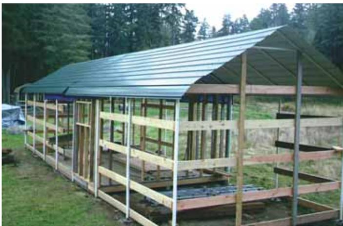
Stewart Kunkel used carport parts to provide the roof and frame for this 12 by 42-ft. barn. Barn is shown here still under construction.
