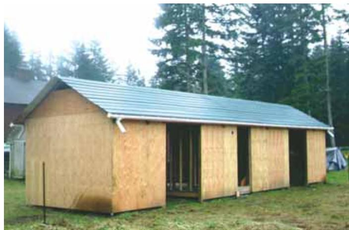
Completed barn has plywood sides and a homemade gutter system.
