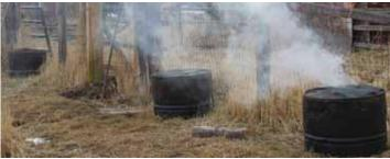
Barrel "ovens" provide a quick and safe way to dig post holes in frozen ground, containing the fire over each post hole spot.
