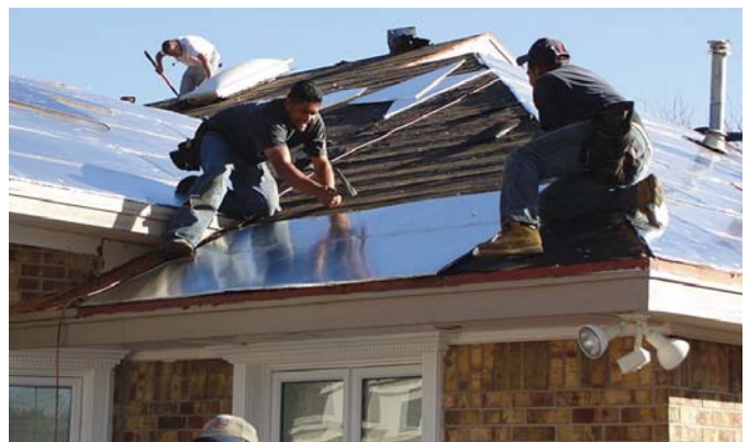
TruProtect is made from laminated layers of reflective aluminum and corrugated board. The 4 by 8-ft. sheets create an energy-saving radiant barrier on roofs.
