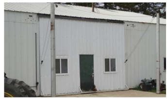
Virgil Poock replaced the worn out door on his shop with a flat panel that has walk- In the closed position, walk-through door and windows result in easier access and bet-
