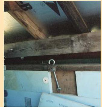
To roll roof open, Padgett folds out and locks triangle braces that bolt to outside wall (left). Then he removes 3 U-hooks from eye bolts screwed into roof.
