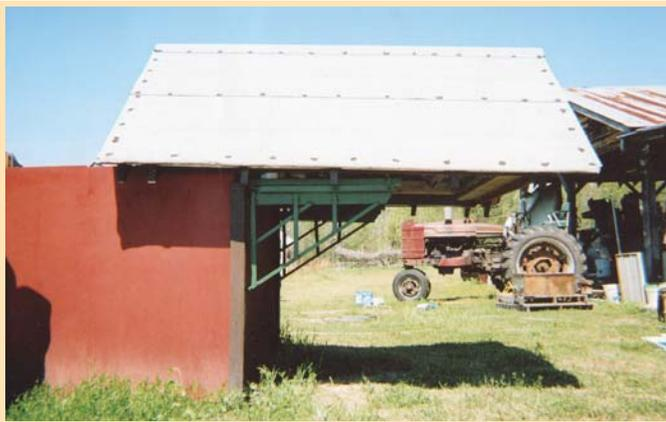
Rolling roof on well house allows James Padgett to pull up a bad well without having to tear the roof off.
