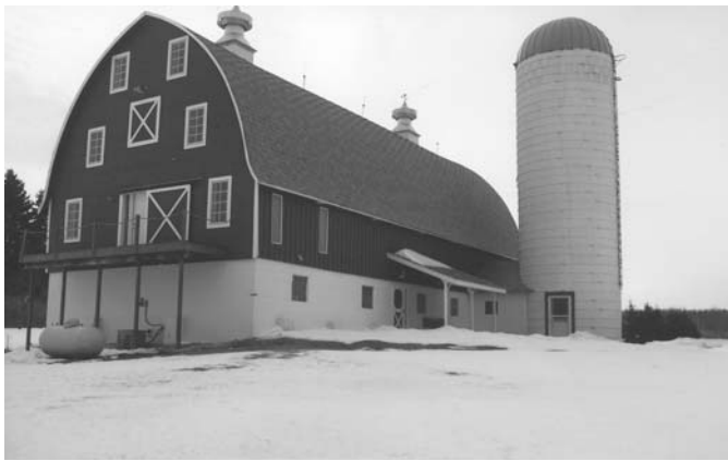
Mike Nistler remodeled this 14 by 40-ft. silo to create a comfortable 4-level hangout for family and friends. Note door cut into side of silo.
