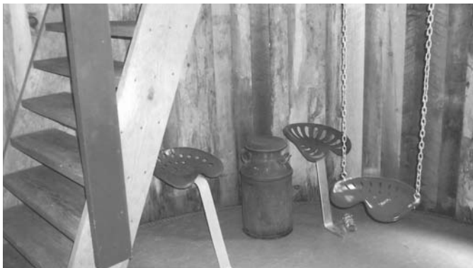
Because of the silo's small diameter, the 25-degree, ladder-like stairs between floors are very steep.
