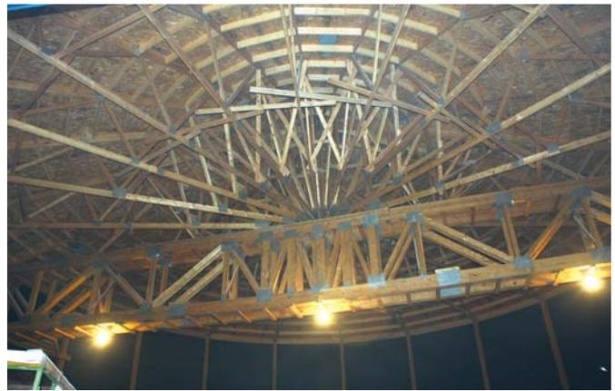
He and a structural engineer came up with a plan for 22 rafters that join at the center, providing a clear span roof.
