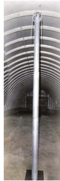
Perforated tube eliminates hot spots and moisture buildup at center of bin. Temperature variations create air flow up the middle and down the sides of bin.
