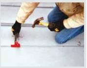
instead of a hammer and nails to do roofing work. Not only does it save time, but the screws hold better and there's no mashed fingers from driving nails.
