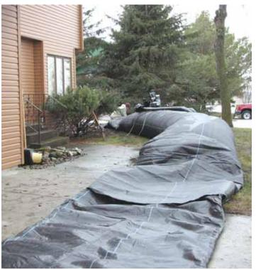
Photo shows Thomas's Aqua Dam being set up around his house. Two sections are connected together. One is filled with water and the other rolled out and ready to fill.
