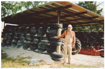
Shed is open in front with 7-ft. high "tire walls" all around. The metal roof is supported by a steel frame that also helps anchor the tire walls. By Bill Gergen, Senior Editor
