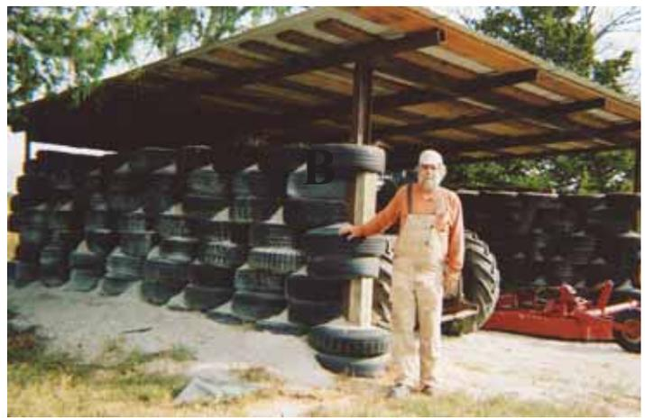
Shed is open in front with 7-ft. high "tire walls" all around. The metal roof is supported by a steel frame that also helps anchor the tire walls.
