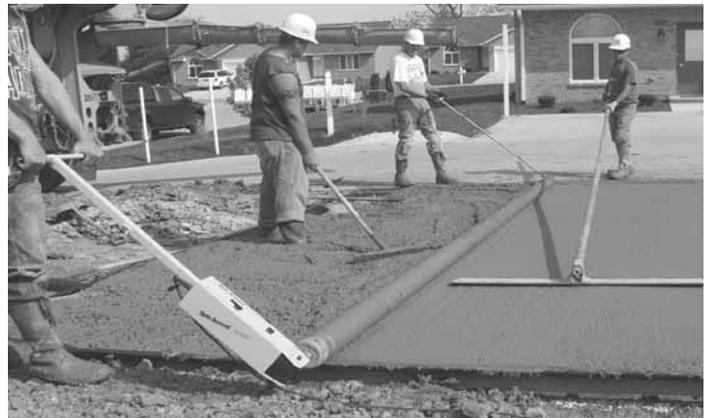
Spin Screed engineers have developed a "Gutter Builder" screed that can be used to build drive over curb and gutters and valley pans in a single pass.
