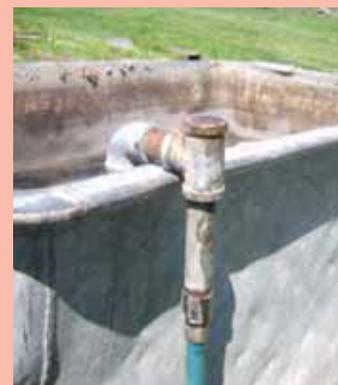
Welding the broken "T" on hose holder accidentally left a small hole that water spouts out of.
