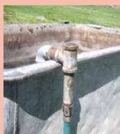
Welding the broken "T" on hose holder accidentally left a small hole that water
