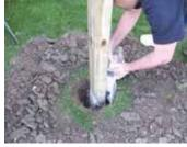
Two-part bag has a different liquid component in each part (left). When mixed together, the 2 liquids form an expanding composite that quickly backfills a post.
