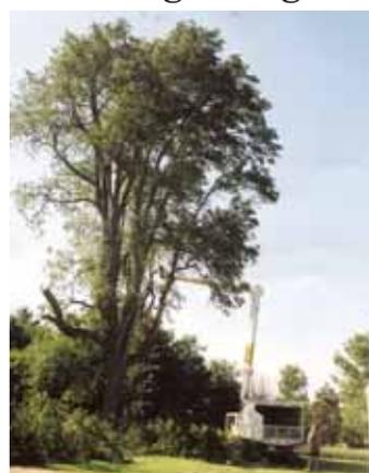
Boom truck is used to install lightning rod near treetop.
