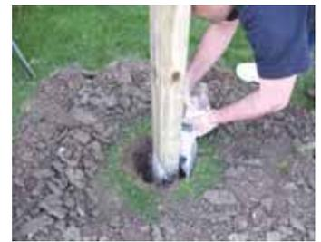
Two-part bag has a different liquid component in each part (left). When mixed together, the 2 liquids form an expanding composite that quickly backfills a post.
