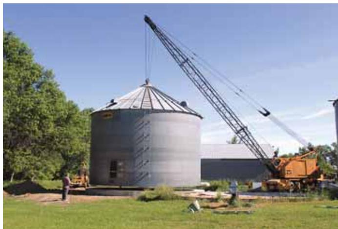
Jerry Kloos, Farmers Cooperative Association in Minneota, Minn., oversees moving a grain bin from an old foundation to a new concrete pad near Canby, Minn. The bin was moved by Kockelman Construction, Inc. of Canby. Replacing broken foundations and moving bins offers a good way to maximize investments. The process, however, takes experience and time to complete correctly.
