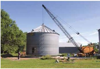
Jerry Kloos, Farmers Cooperative Association in Minneota, Minn., oversees moving a grain bin from an old foundation to a new concrete pad near Canby, Minn. The bin was moved by Kockelman Construction, Inc. of Canby. Replacing broken foundations and moving bins offers a good way to maximize investments. The process, however, takes experience and time to complete correctly.
