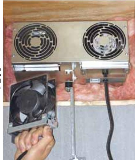
Reversible dual fan module can be set to bring in fresh air, and exhaust stale air.
