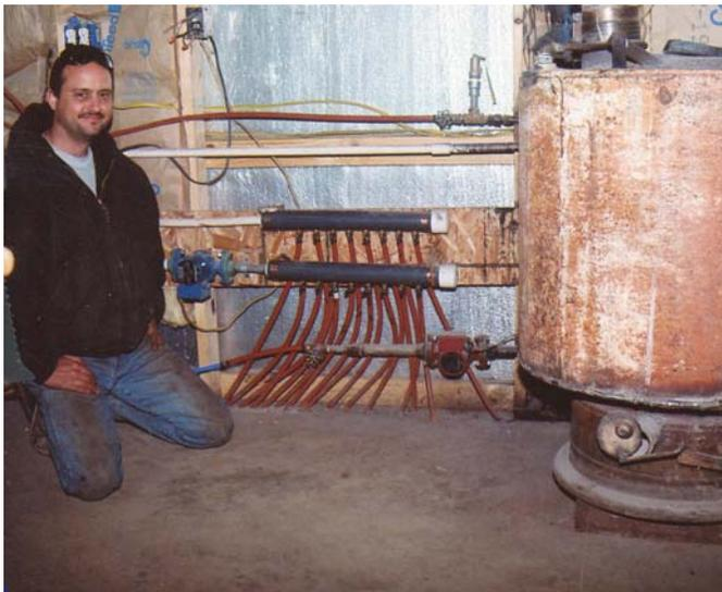
**Bob Bugger welded truck wheels together to build his own shop furnace. A heated anti-freeze mixture is pumped through plastic tubing under his shop's floor.**
