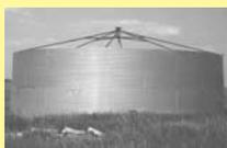
**Low-Cost Temporary Bin (Vol. 23, No. 4)** - Jim Noram spent \$600 to put up a bin with no floor or roof. It measured 36 ft. in dia. and held 13,000 bu.
