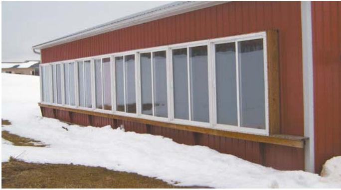
Steven Ratliff used old sliding glass doors to build solar collector panels. They cover the south wall of his 30 by 60-ft. machine shop.
