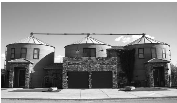
Don and Carolyn Riedlinger moved onto a 9-acre home site and made a home out of three connected, 28-ft. dia. grain bins.
