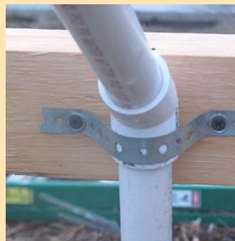
Plants grow in high tunnels into late fall (top). A 20-ft. long pvc pipe fits into coupling on sidewall (left above) and goes up to building's 2 by 4 ridgepole, then slips into another coupling on opposite wall. Side curtains raise up for ventilation.
