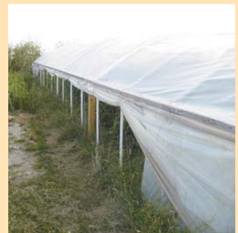
Plants grow in high tunnels into late fall (top). A 20-ft. long pvc pipe fits into coupling on sidewall (left above) and goes up to building's 2 by 4 ridgepole, then slips into another coupling on opposite wall. Side curtains raise up for ventilation.
