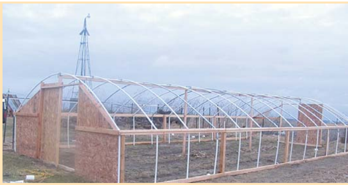
Market gardener Jay Sleichter couldn't justify the cost of a commercial-built "high tunnel" so he built his own using wood and 1-in. pvc pipe.
