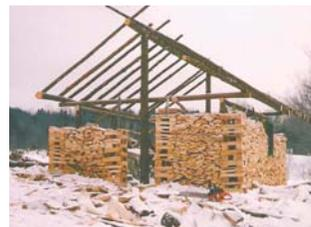
To build cabin's walls he simply stacked 16-in. lengths of slabwood on top of each other, using an interlocking technique at each corner.
