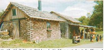
Alec Alberti built this pair of "slabwood cabins" from mortarless stacks of firewood. Roof is independently supported by end poles.
