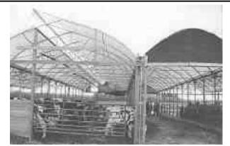
One of the latest designs in low-cost structures comes from Harnois. The company has designed a way to "gang" the shelters together side-by-side with rain gutters running between buildings.
