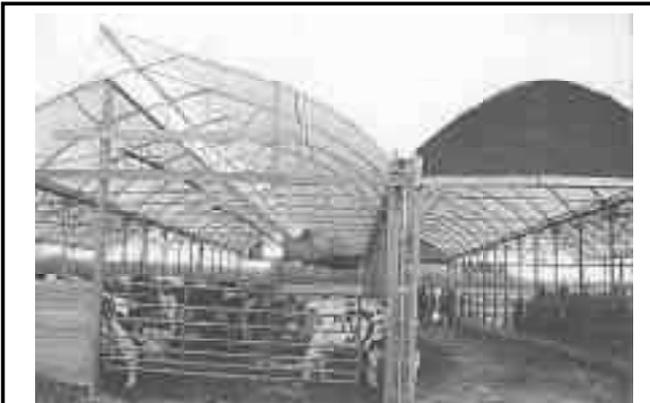
One of the latest designs in low-cost structures comes from Harnois. The company has designed a way to "gang" the shelters together side-by-side with rain gutters running between buildings.
