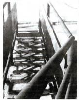
trying to turn around. Posts on either side of the chute are 4 1/2-in. in dia. Side rails on the chute and fence around the holding pen are made from 3 1/2 in. dia. oil field pipe, with rails made from 2 1/4-in. dia. pipe and 3/4-in. dia. sucker rod.
