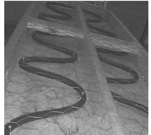
Compost-heated water runs through lengths of insulated hose under growing tables in greenhouse.
