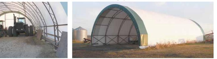
Silver Stream's new free-standing shelters are available with steel truss hoops, as shown in this new building.
