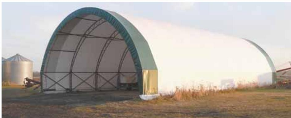
Silver Stream's new free-standing shelters are available with steel truss hoops, as shown in this new building.
