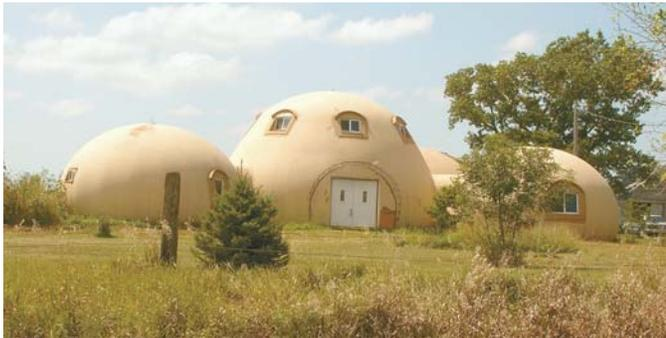
"Home domes" were created using airforms – big polyvinyl balloon-like shells inflated with air. Main dome is 32 ft. in dia. by 20 1/2 ft. tall.
