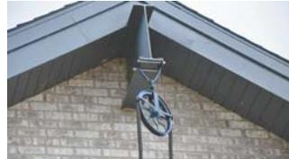
Pulley mounted on 24-in. I-beam over garage (left) comes in handy for unloading heavy cargo. Kitchen light was made from an old scissor-type casket carrier.
